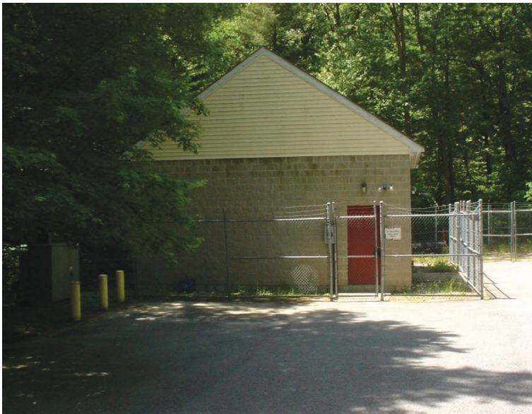
Glen Street Pump Station
